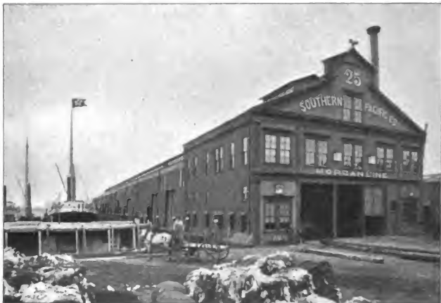
SOUTHERN PACIFIC COMPANY -- "MORGAN LINE," -- PIER 25, NORTH RIVER.
